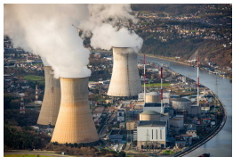
The Tihange nuclear power plant in Belgium
