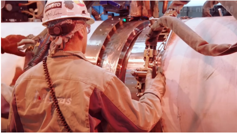
Fortuna welder positioning the automatic welding machine
