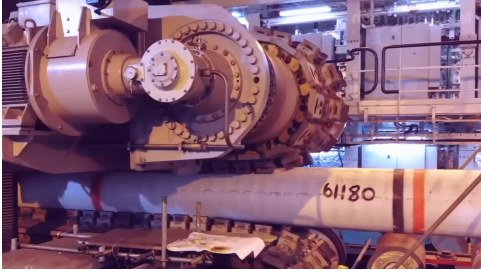
The pipeline passing the hydraulic tensioner
